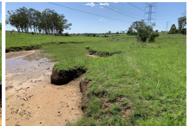
Facing downstream – dry dam
