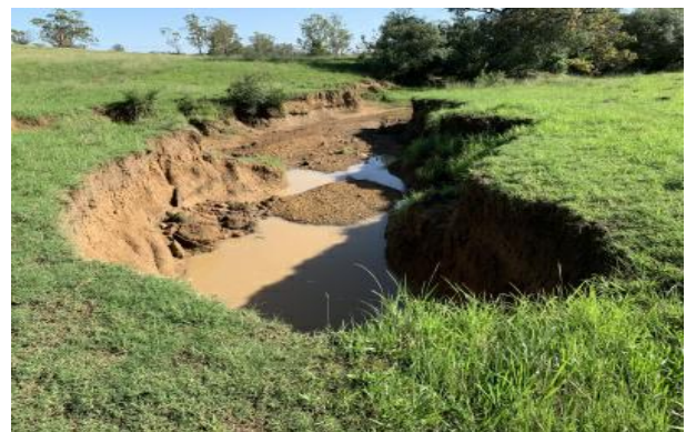
Channel joins dam at large eroded feature
